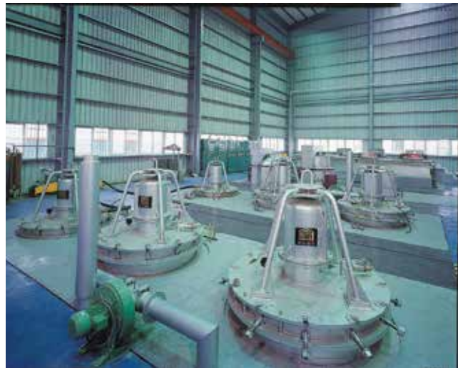
Quench & Tempered Facility
